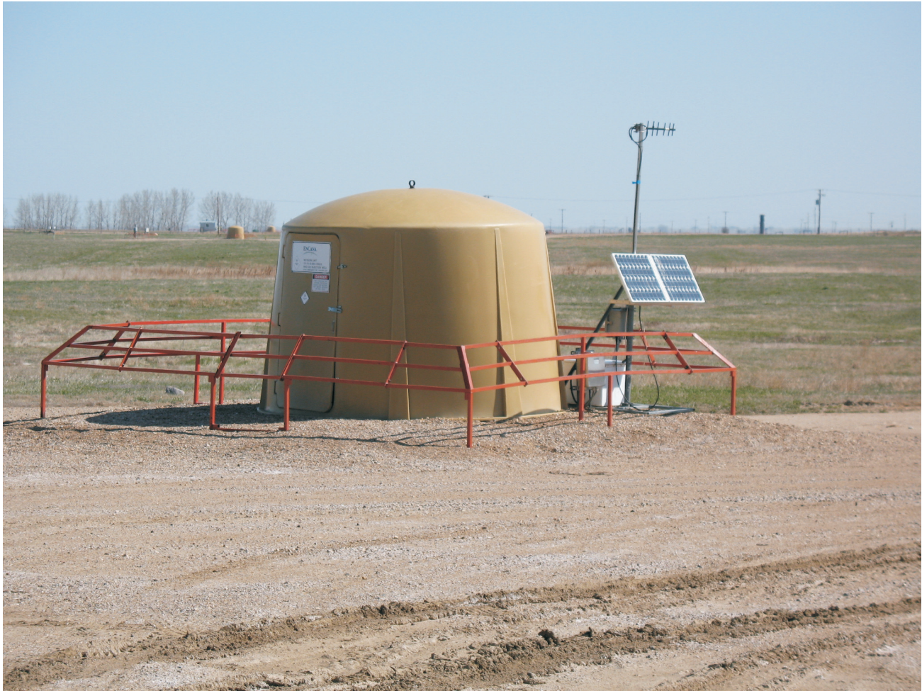
CO 2 injection wells are generally small and have little impact on surrounding areas, as shown in this picture of a CO 2 injection well in Canada.
