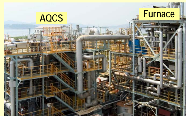
1.5MWth test facility
