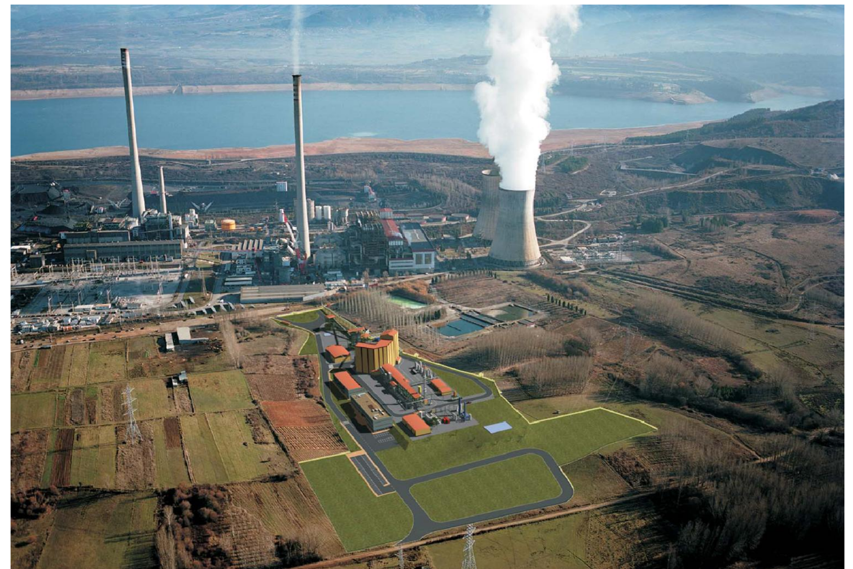
CIUDEN CCS large scale test Platform which is close to Compostilla Power station.
