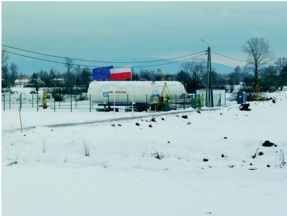
CO2 being stored in tanks for injection at the RECOPOL field test site in Poland
