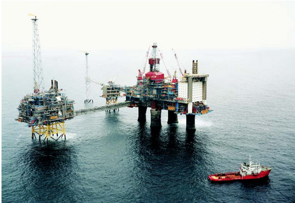
Sleipner production platform. (Courtesy of Statoil)
